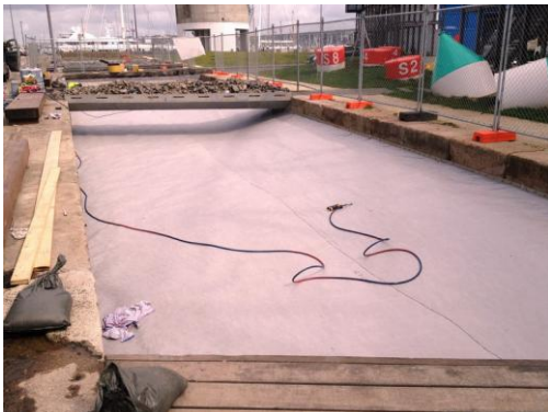
Application of geotextile
