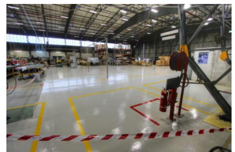
After: The completed hangar floor
