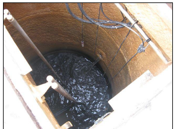
Finished live wet well
