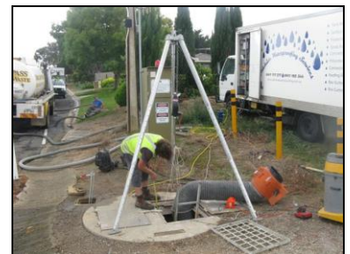
Confined space and limited access
