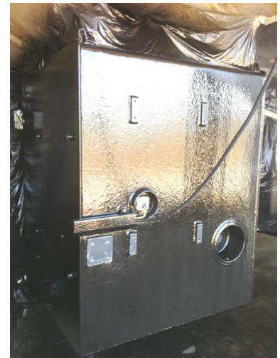
Diesel Tank Coating
