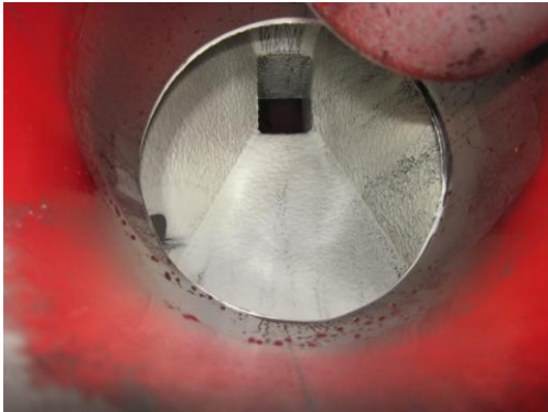
Cyclone overflow box after 12 months
